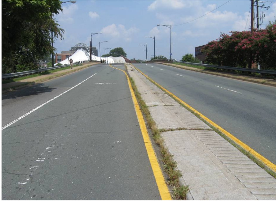
ROADWAY LOOKING NORTH
