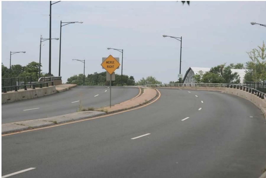
ROADWAY LOOKING SOUTH
